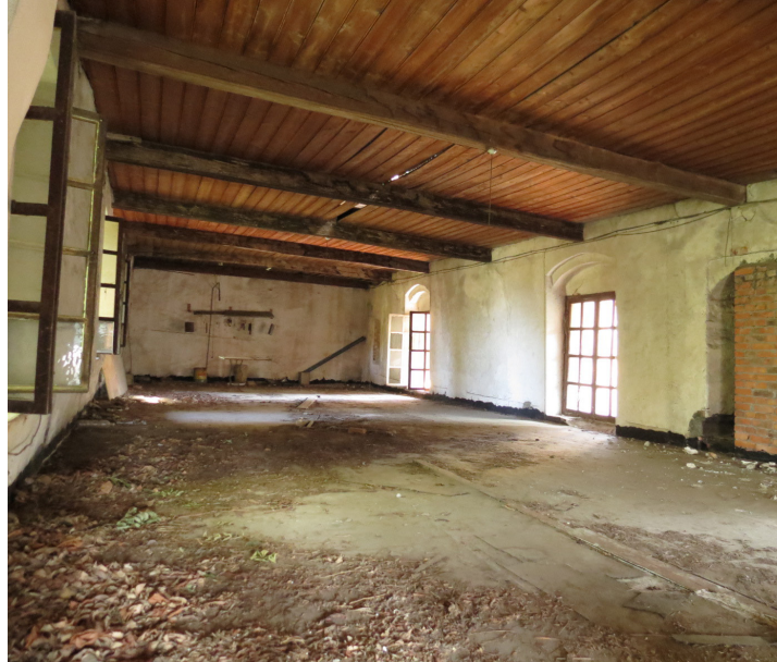
5 Picture of the attic
