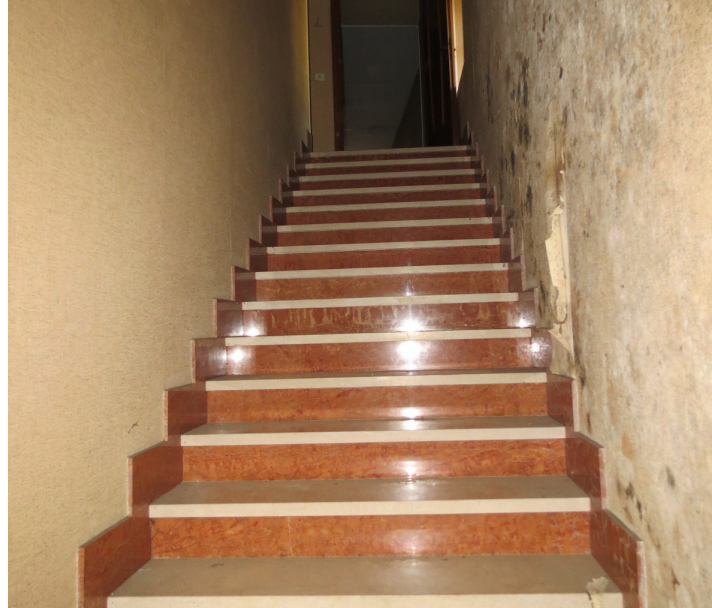
7 Picture of the stairs between the ground and the first floor
