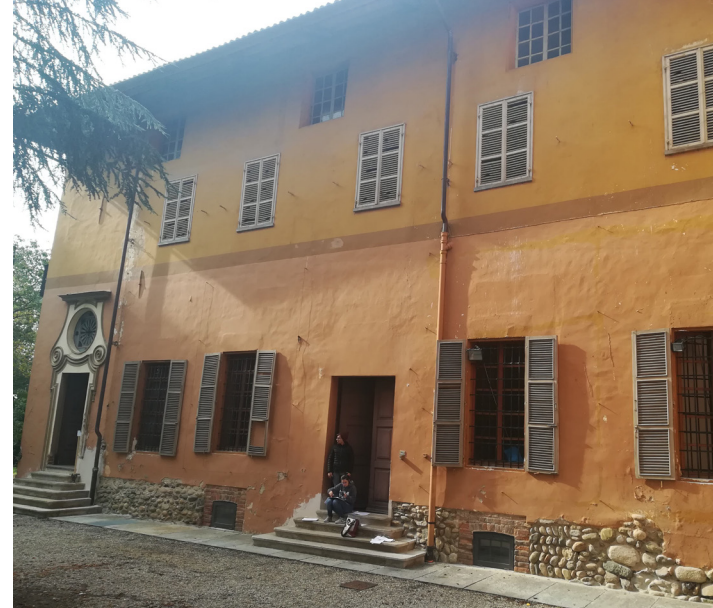
9 Picture of the south facade
