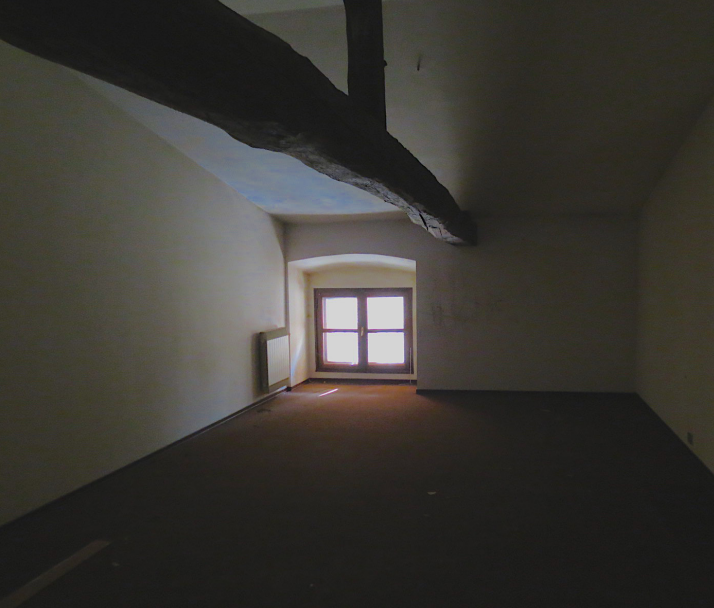
3 Picture of the attic truss
