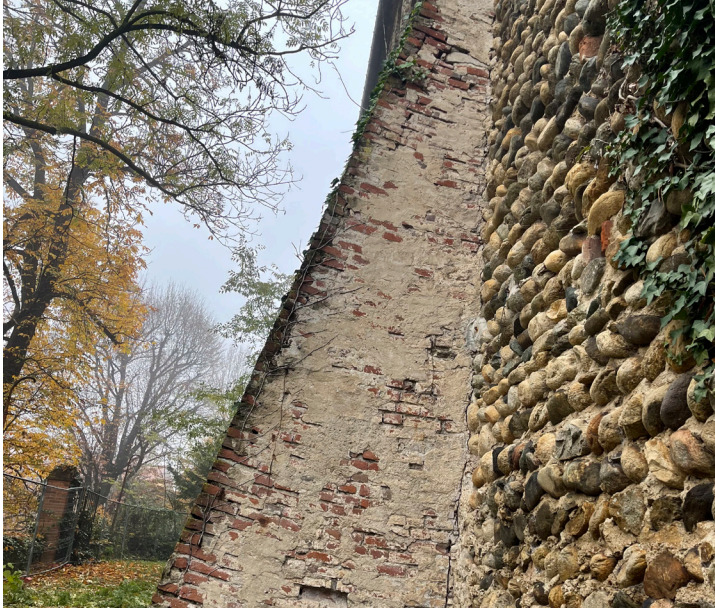
4 Picture of the brick buttress
