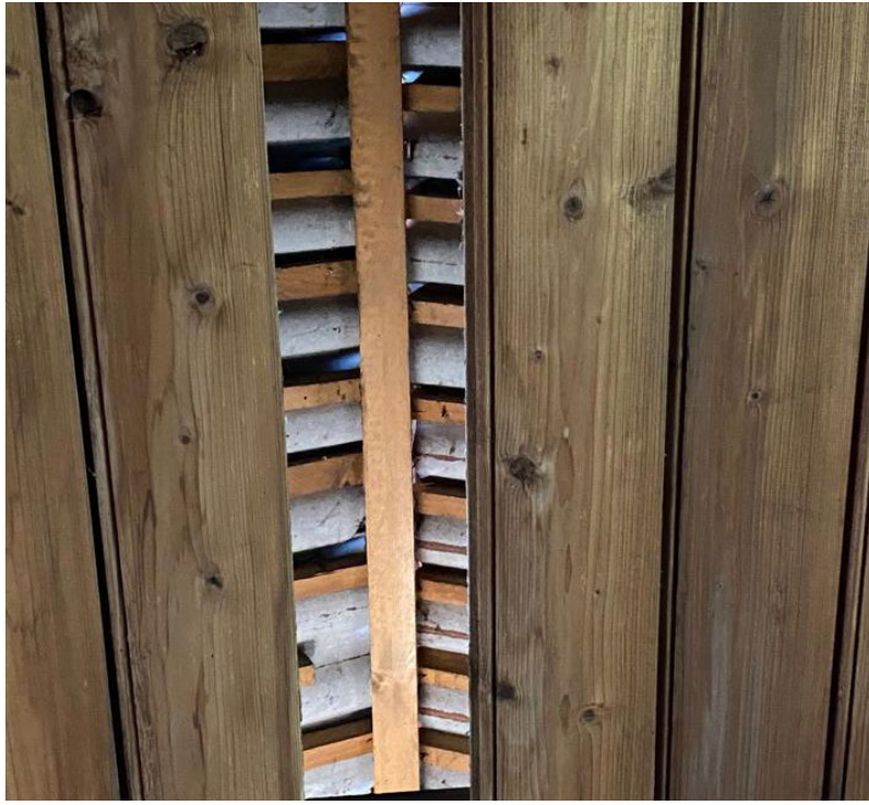
c Truss of the eighteenth-century sleeve seen from the fissures of the beams that currently cover it
